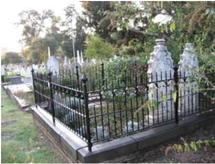
Carlile Fence - after repair
